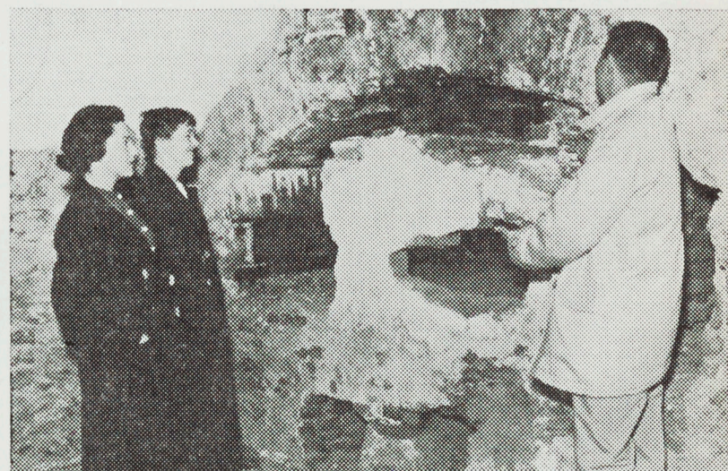
Moravian students Betty Ann Dickman, Jane Albrecht, and Bill Pfeiffer observe newly-discovered colonial bake oven at Brethren's House, South Campus. It is believed that after a fire had sufficiently heated the internal structure of the oven, the fire and ashes were removed to make way for the dough. The bricks stayed hot long enough to properly bake the bread.
